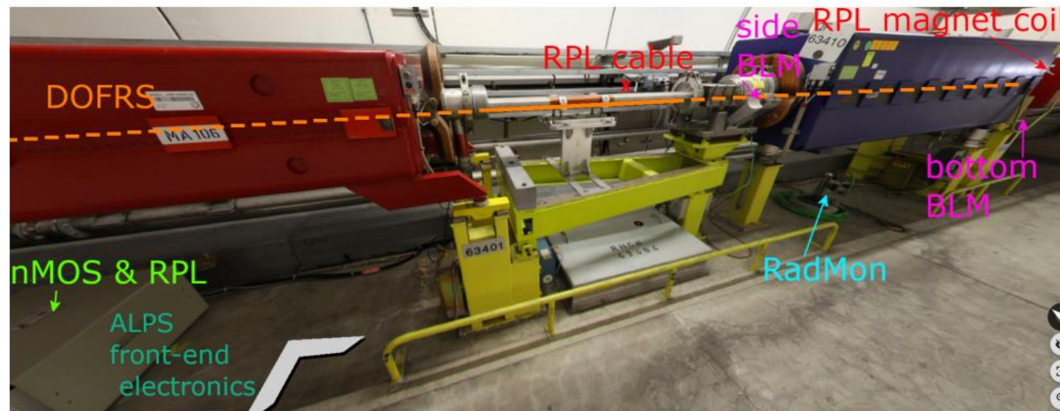
Fig. 4. Standard positions of the radiation sensors in the SPS arc sections, with the electronic rack of the ALPS system (with nMOS dosimeter on top, \sim 0.9 m distance from the beamline), directly exposed to the mixed-field radiation. Behind the magnets, at the cable tray ( \sim 1.3 m distance), as of 2021 the DOFRS monitor is installed. Before 2021, the Total Ionizing Dose was assessed by the RPL dosimeters ( \sim 1 m distance), in each arc half-period one installed at the cable tray, and one at the magnet coil. Each arc half-period contains one Beam Loss Monitor, installed either at the side of the beamline ( \sim 30 cm distance) or under the first dipole magnet, as in the presented location. Additionally, in some half-periods RadMons are deployed under the magnets.
