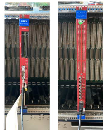
TDC and VME bridge
