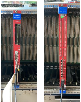
TDC and VME bridge
