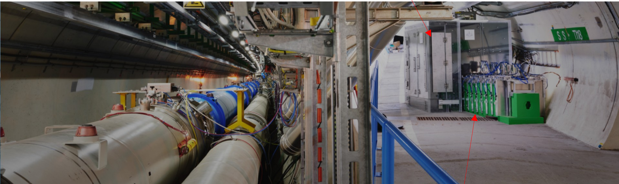
SND@LHC view, installed close to LHC machine
