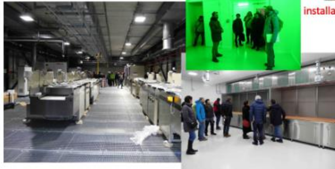
Construction of the new workshop's building
