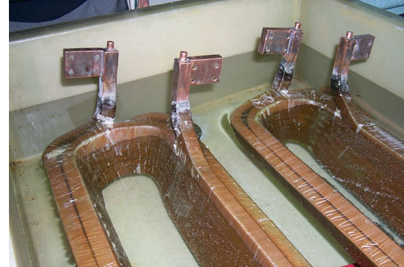
coil electrical test (under water !)
