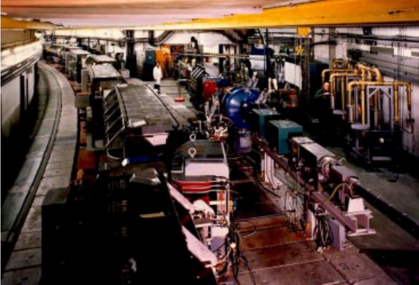
Fig. 12.1: View inside the CERN-PS tunnel (Photograph: CERN).
