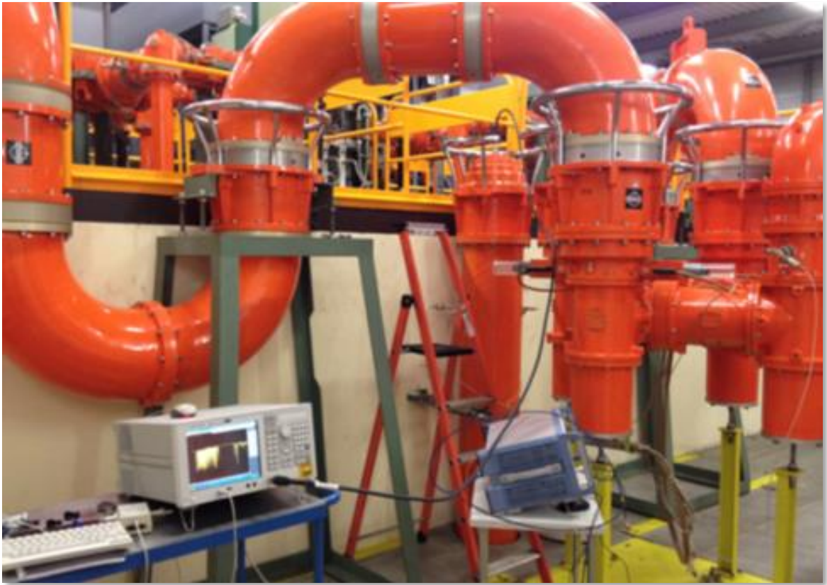
SPS 200 MHz cavity feeder line.
