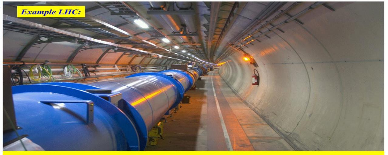
7000 GeV Proton storage ring dipole magnets N = 1232 l = 15 m q = +1 e
