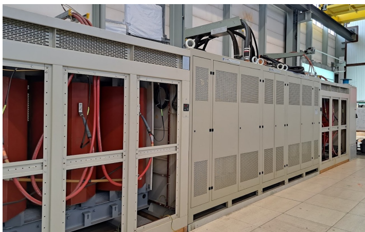
RPTE – LHC main dipoles 13 kA / 190 V, 2-quadrant
