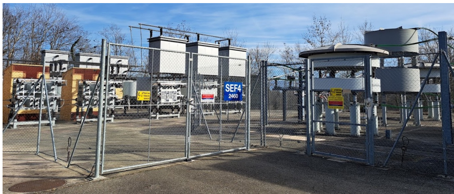
Static VAR Compensator (SVC) – at LHC P2, P4, P6, P8
