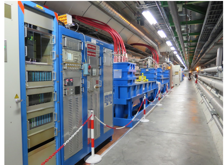
Service area near one of the LHC access points, CERN
