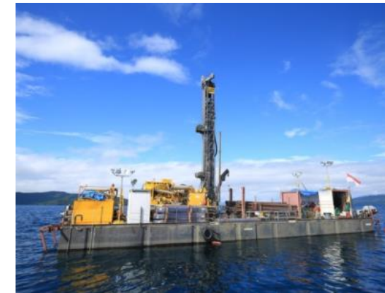
Drilling works on the lake
