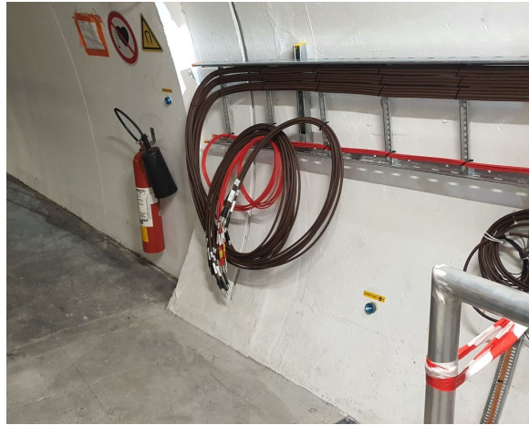
August: Cabling installed by cern
