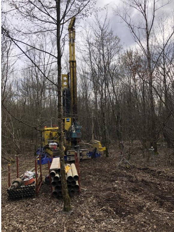
➤ Drilling machine in place
