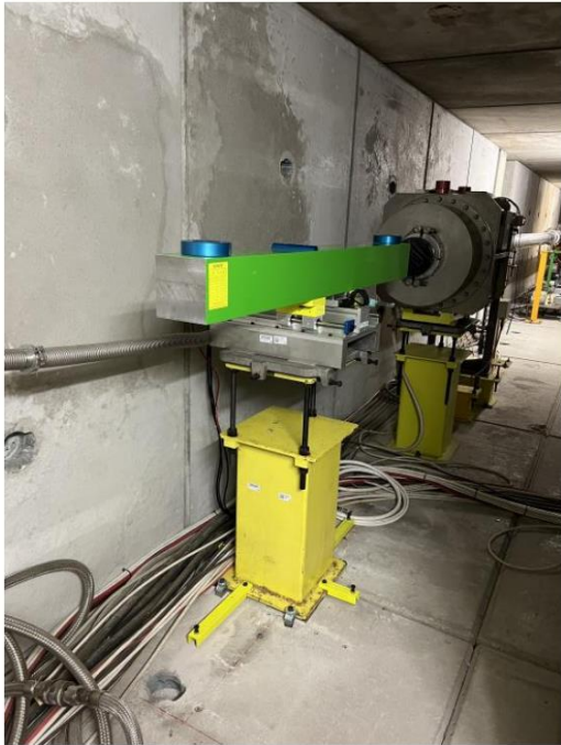
Figure 10 – Installed XCIO on the line.
