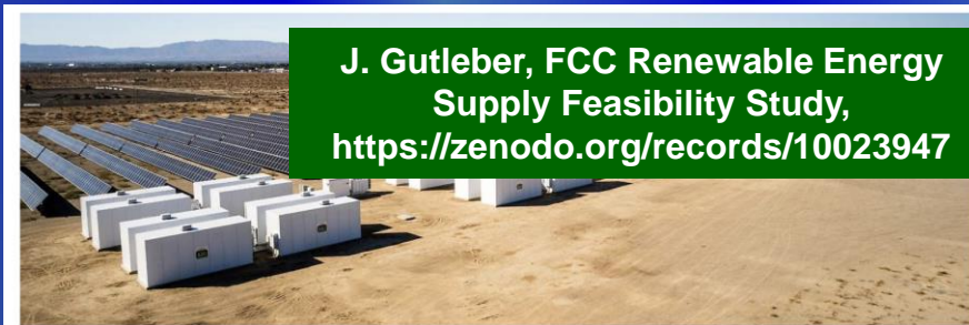
Figure 7: A single 25 MWh energy storage unit (white containers) built from used electric car batteries, deployed for a PV energy plant in Lancaster, CA (south of Los Angeles, US) put in operate by B2U Storage Solutions in early 2023. Capacities of new systems are increasing fast. A 260 MWh 25 is by now being commissioned and today's largest systems in the range of 1 400 MWh are being extended to 3 000 MWh 26 .
