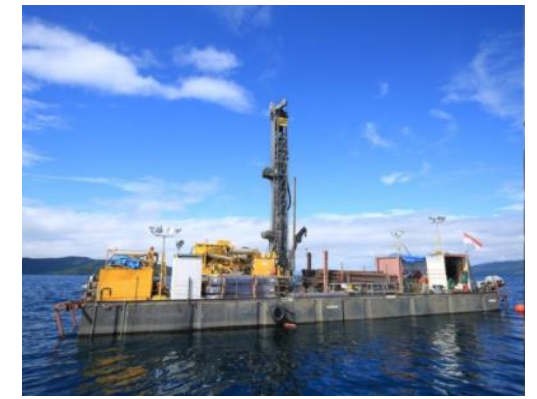
Drilling work on the lake
