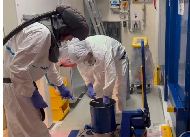
Disconnecting small and large drums
