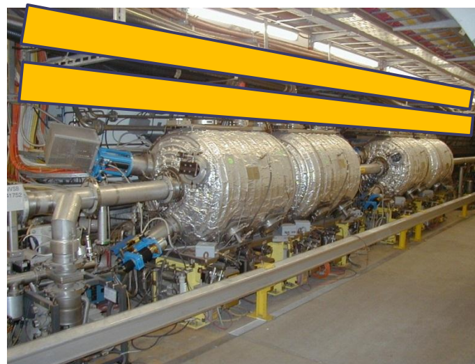
Tunnel between Coldex (left) and ECX4 (right) (ex-SWC100)
