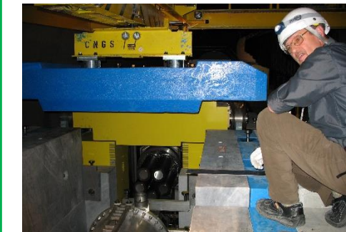
Installation of horn roof shielding
