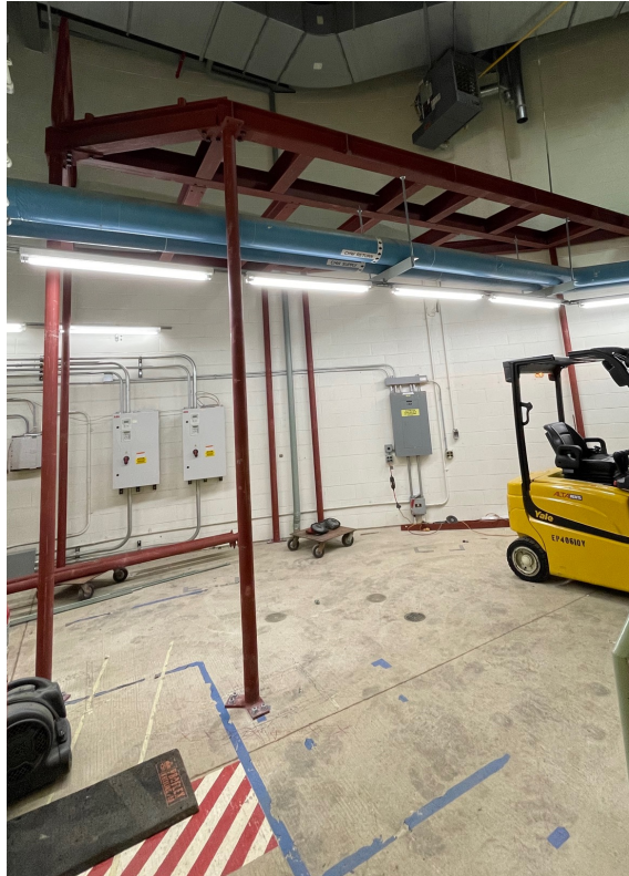
Construction started in 2023.
