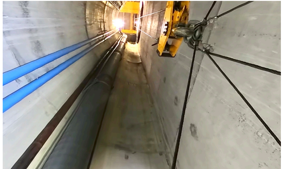
View from camera on top of personnel basket.
