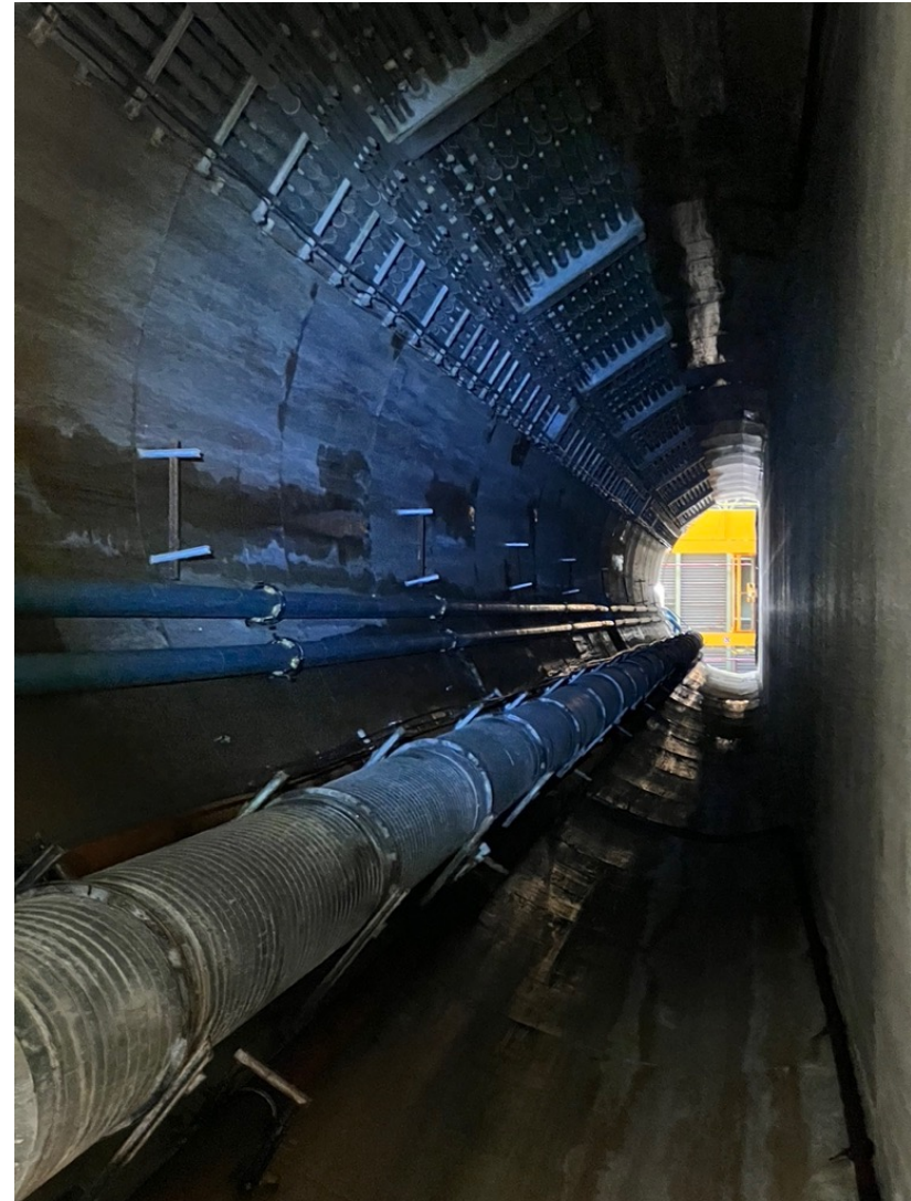
View looking up from inside shaft.
