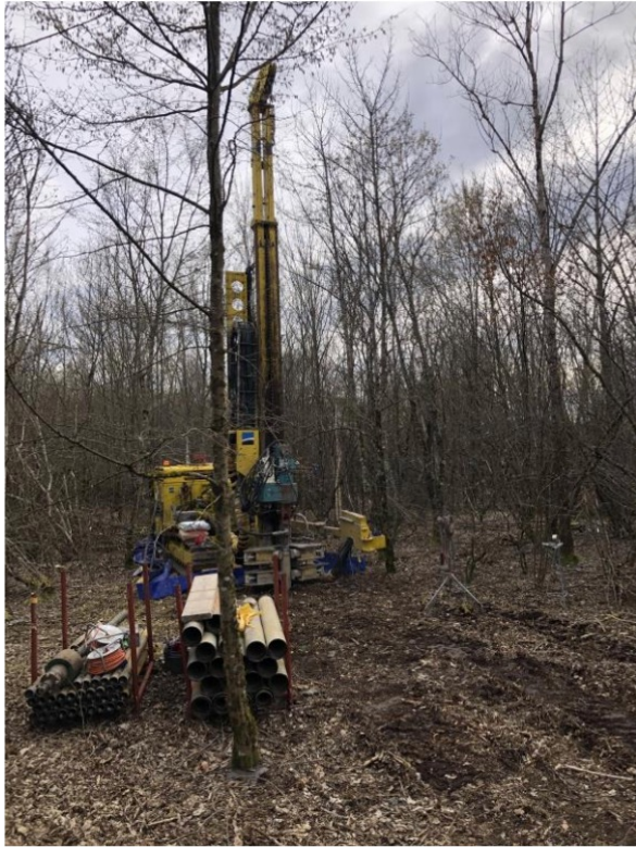
➤ Drilling machine in place
