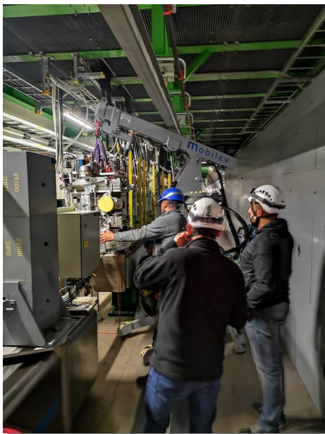
Removal of two ATLAS-ALFA Roman Pot stations after high- \beta run 2023
