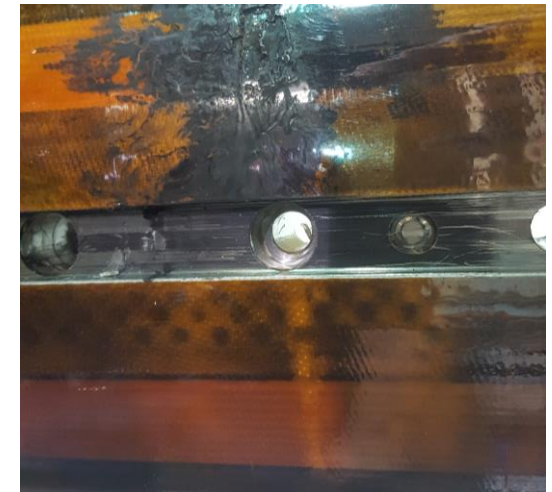
Result of electrical short circuit quench heater to coil in a Nb 3 Sn coil
