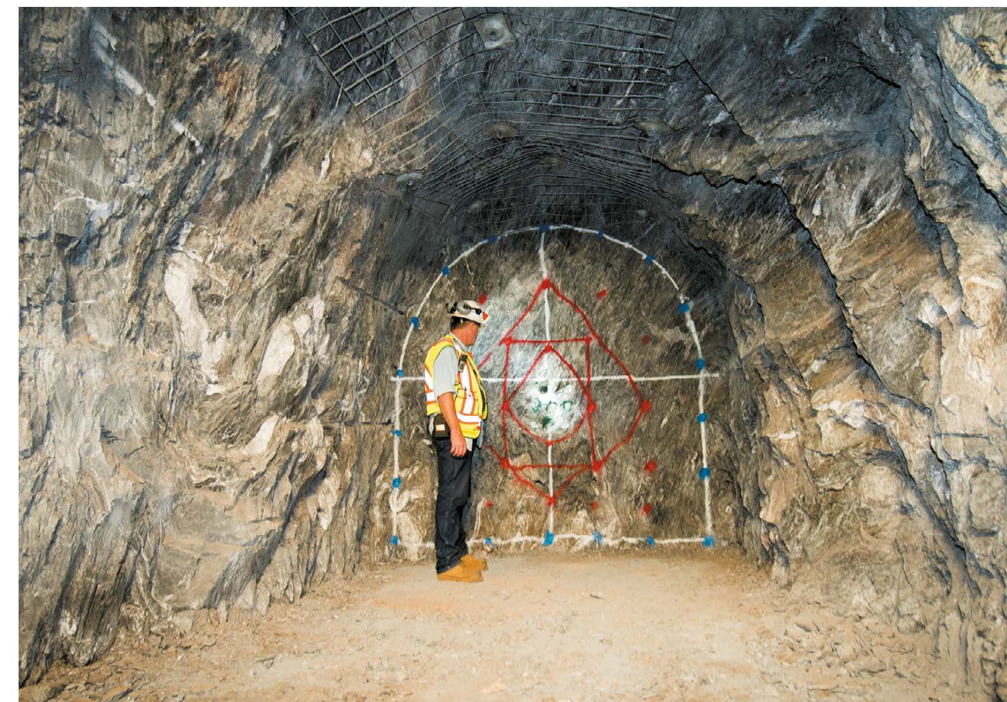
An underground test blast area for the DUNE neutrino experiment in Lead, South Dakota.
