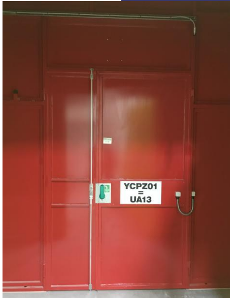
End-of-zone door of the LHC Access Safety System (LASS), for emergency exit at the bottom of PX46 Red in color and including an emergency opening handle on both sides
