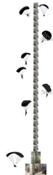
LHC gas system racks: > 500 m
