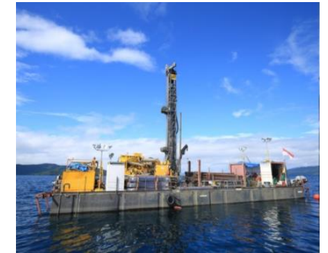
Drilling works on the lake
