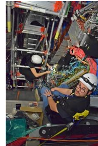
VTRx replacements on NSW rim
