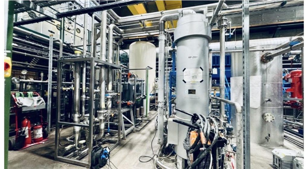
New dryer installation
