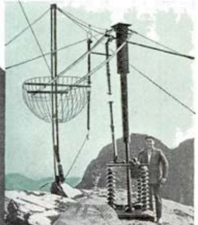
Here is part of the apparatus that was used in the Mt. Generoso tests. This strange network was designed to carry the enormous voltage to the laboratory where the scientists waited in danger of instant death.
