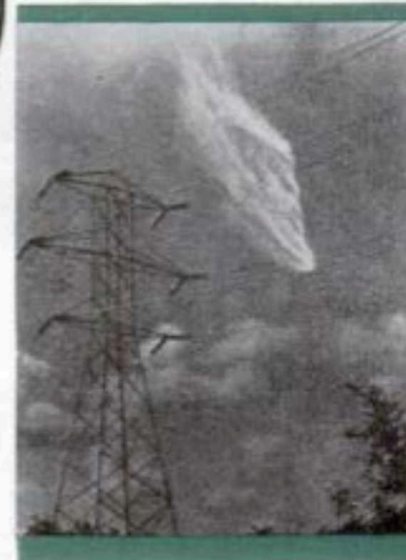
High-voltage currents, knowing no bonds, do strange things. Here is an arc that is leaping between two high-tension wires.
