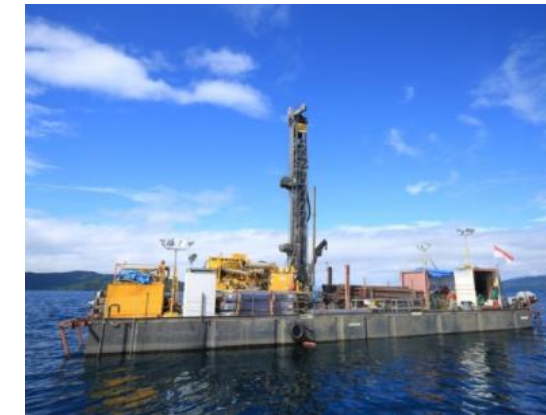
Drilling works on the lake
