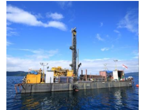
Drilling works on the lake
