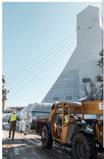
TPC inside inner cryostat vessel (ICV) being transported underground
