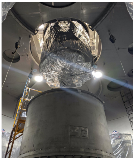
ICV being lowered into the outer vessel inside the water tank
