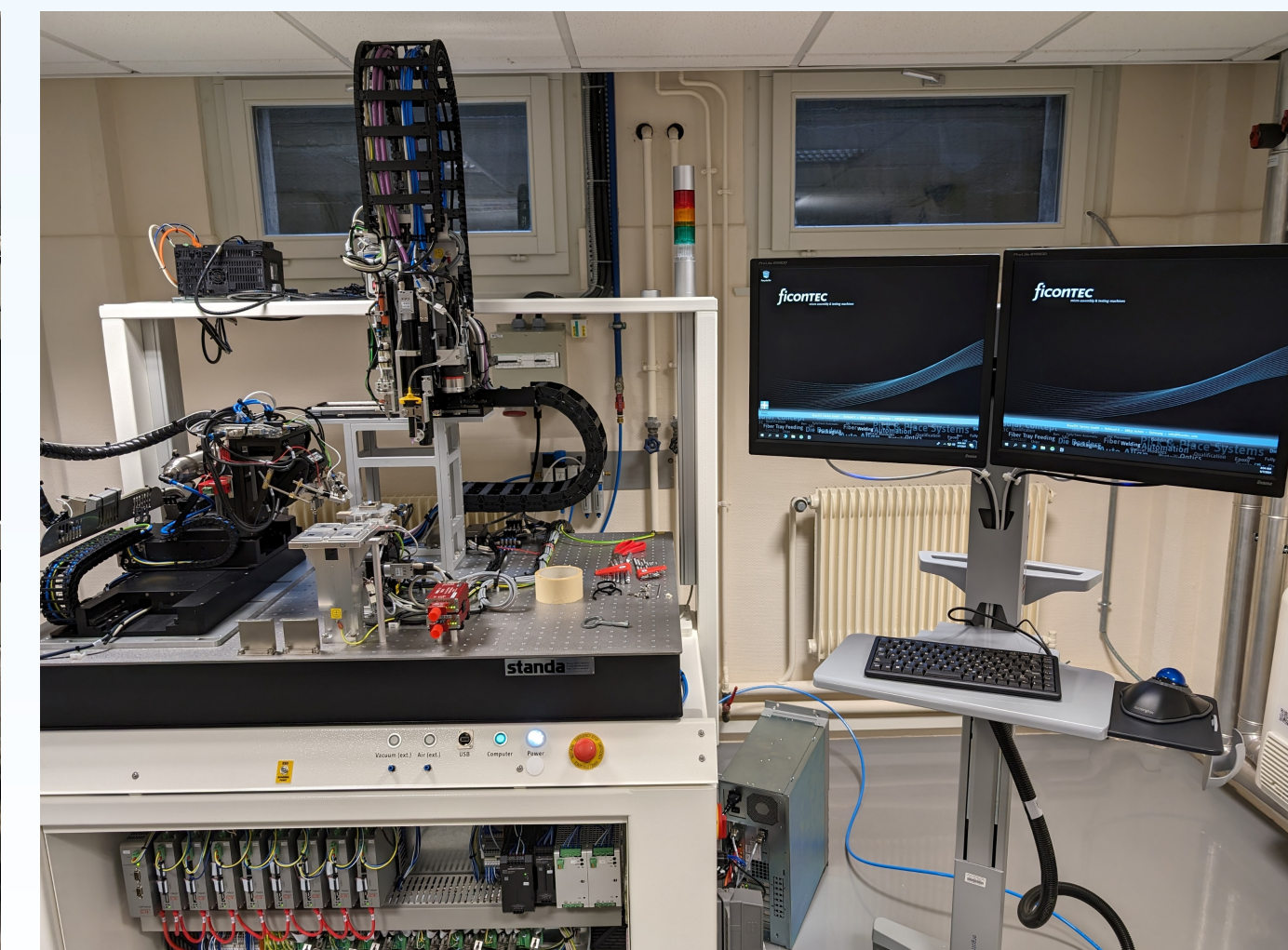
Machine installed in B13
