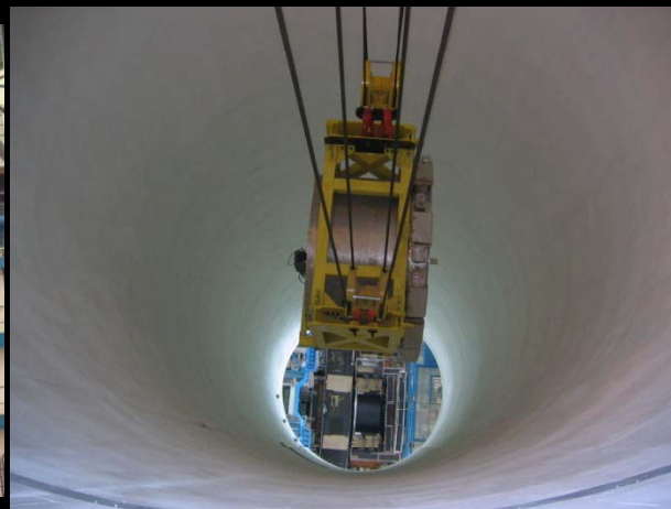
Lowering down the shaft
