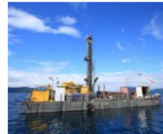
Drilling works on the lake
