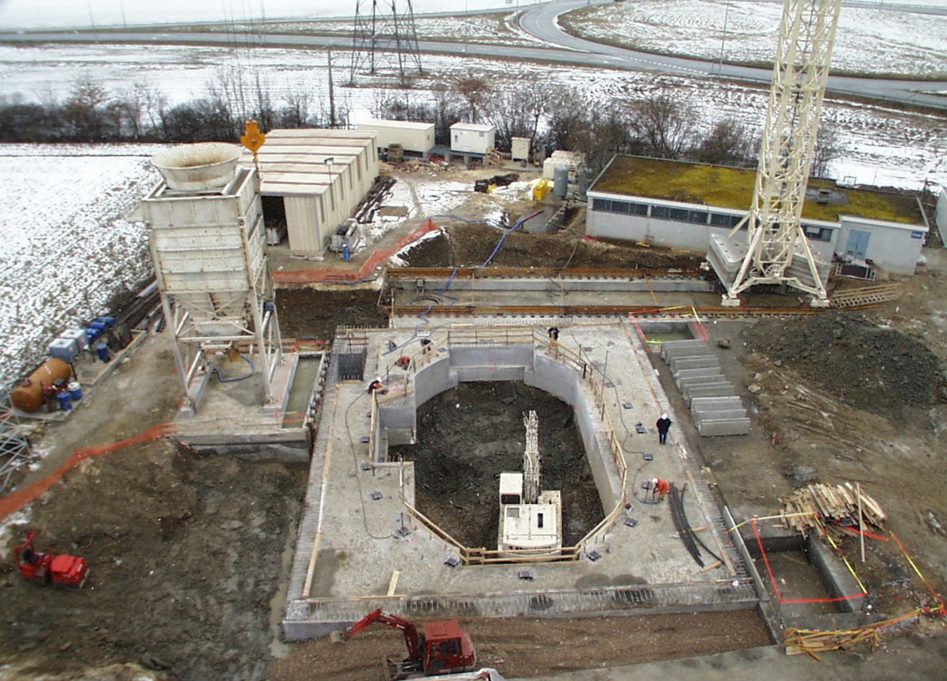
T12 Area - Start of excavation of PMI 2 shaft - February 17, 1999 - CERN ST-CE
