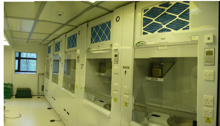
Class 10 000 area (Bio, Photochemical, MEMS, Photolith cabinets)
