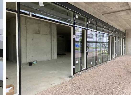
View on the main entrance
