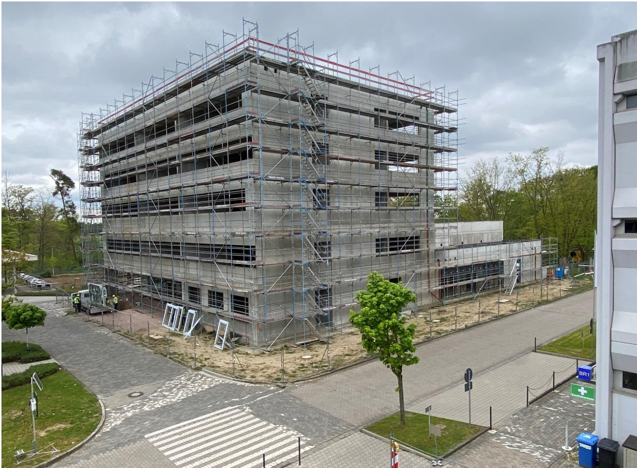
View on the north and south facade
