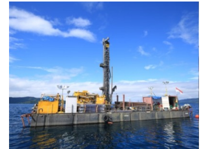
Drilling work on the lake
