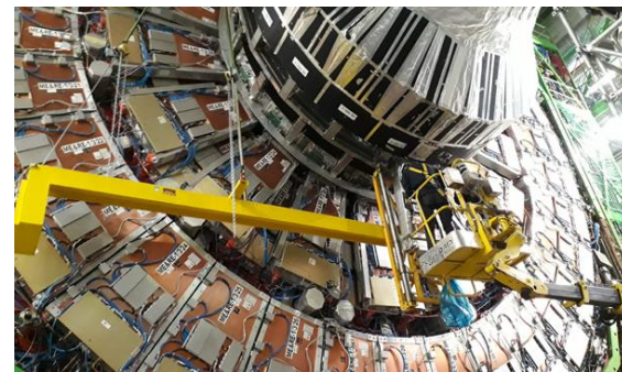
ME1/1 CSC installation
