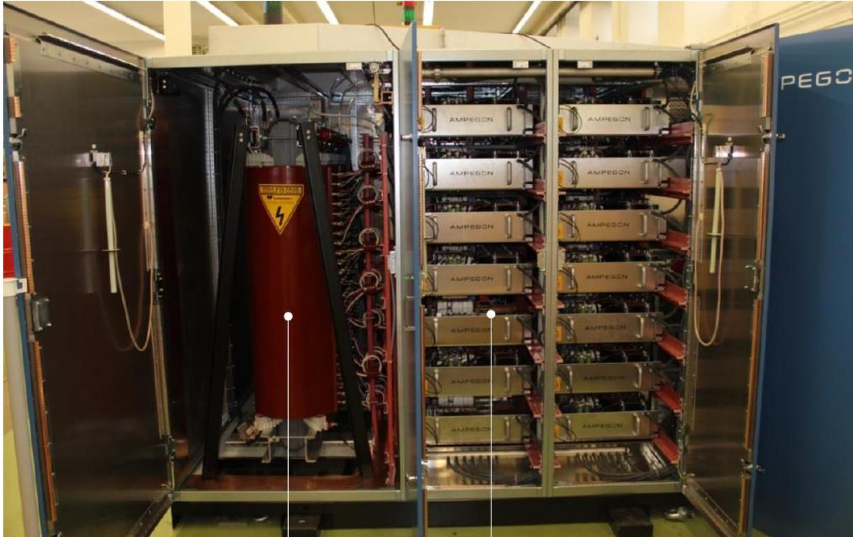
Modules are controlled via PWM principle (*Pulse Width Modulation*)
