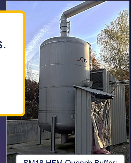
SM18 HFM Quench Buffer: 15 m 3 @ 5 bar @ 5 K
