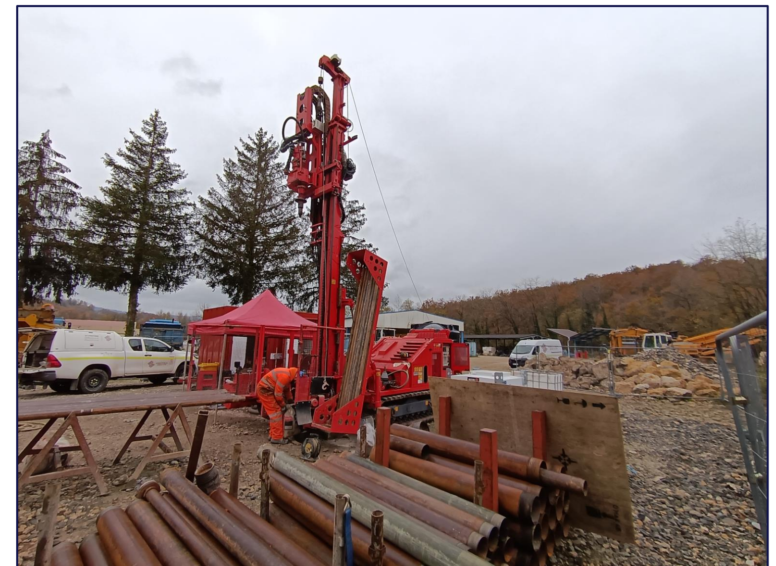
Drilling rig at Usse_2 site
