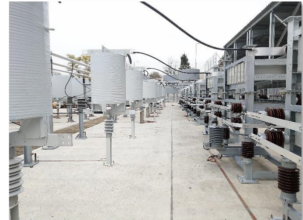
TCR: Thyristor-Controlled Reactor
