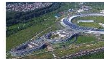
Nov. 3, 2023 Civil Construction for ancillary buildings completed
