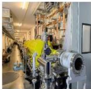
May 12, 2022 The Linac Vacuum-sealing in the tunnel completed
