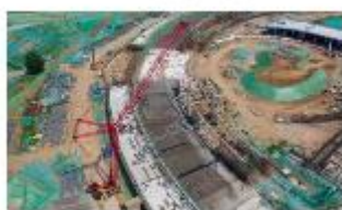
July 1, 2020 The first steel beam was installed
