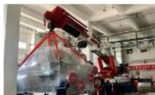
Apr. 13, 2021 Utility installation in NO.2 Hall commenced
