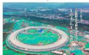
June 27, 2021 Roof-sealing work for the main ring building completed
