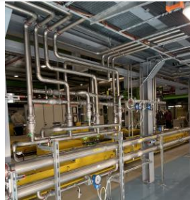
Water-Cooling System (config for HL tested – ECR by L. Tavian )
