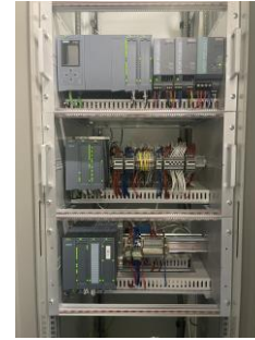
Prototype PICv2 (New PIC for HL-LHC and planned to be deployed in LHC)
