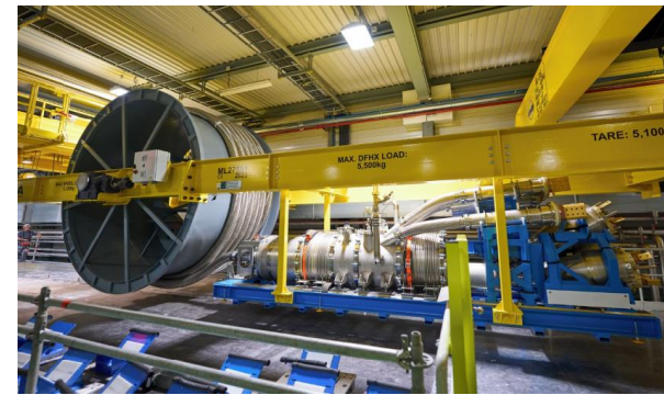
Equipment fixed in secured structure
