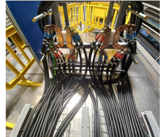
Ultra-flexible class 6 cables
