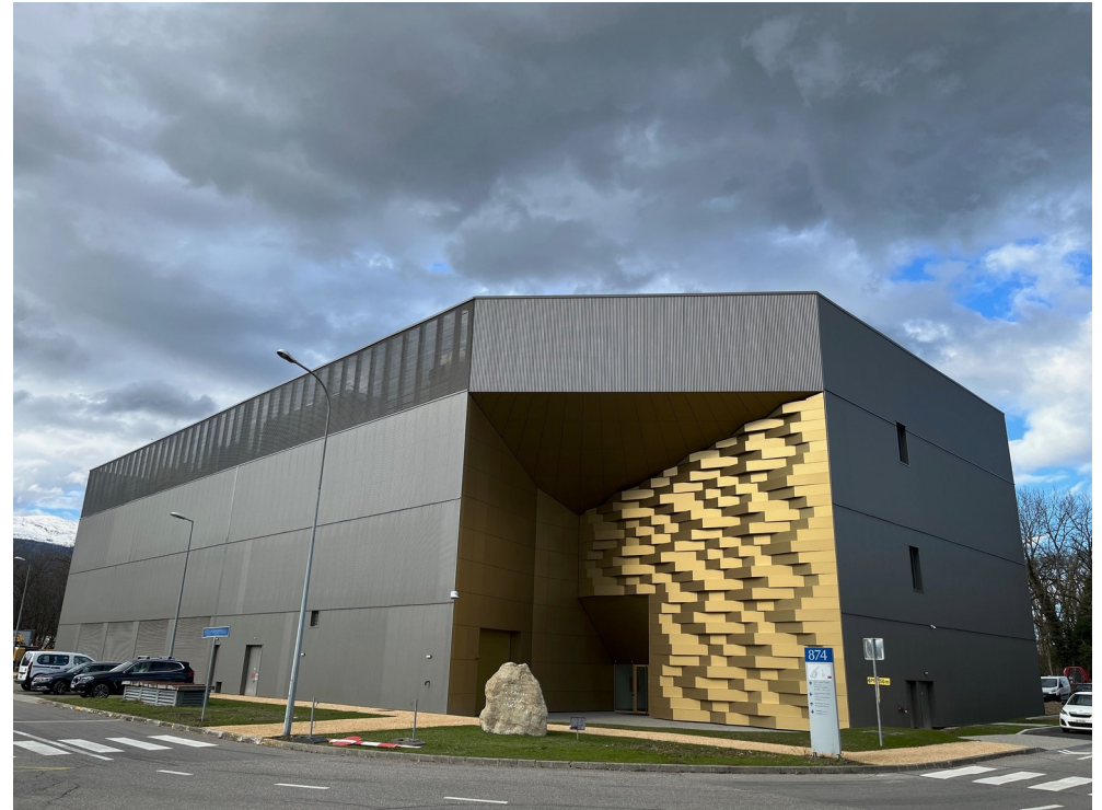
CERN Prevezin Data Centre
