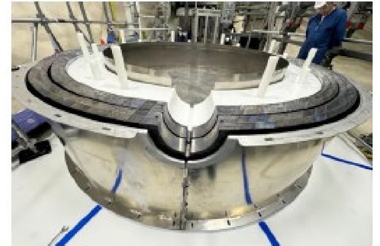
Shield base installation completed
